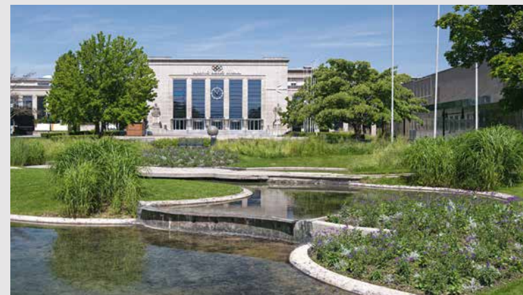
Beaulieu Lausanne set in extensive gardens
